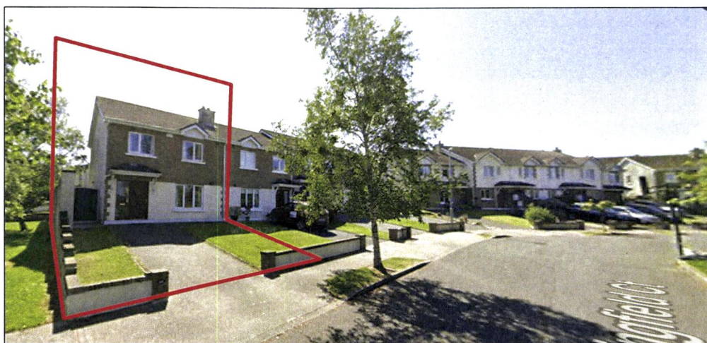
Figure 2: View of 26 Springfield Court
